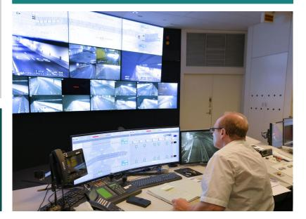
"The installation of new Bosch IP cameras delivers improved performance, as well as onboard analytics that Sydney Harbour Tunnel will use to count vehicles, as well as to deliver an additional layer of fire protection."
